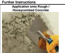
**Finishing Porous Concrete in** Precast Concrete
